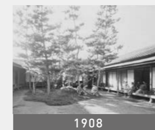
Detached family housing units
